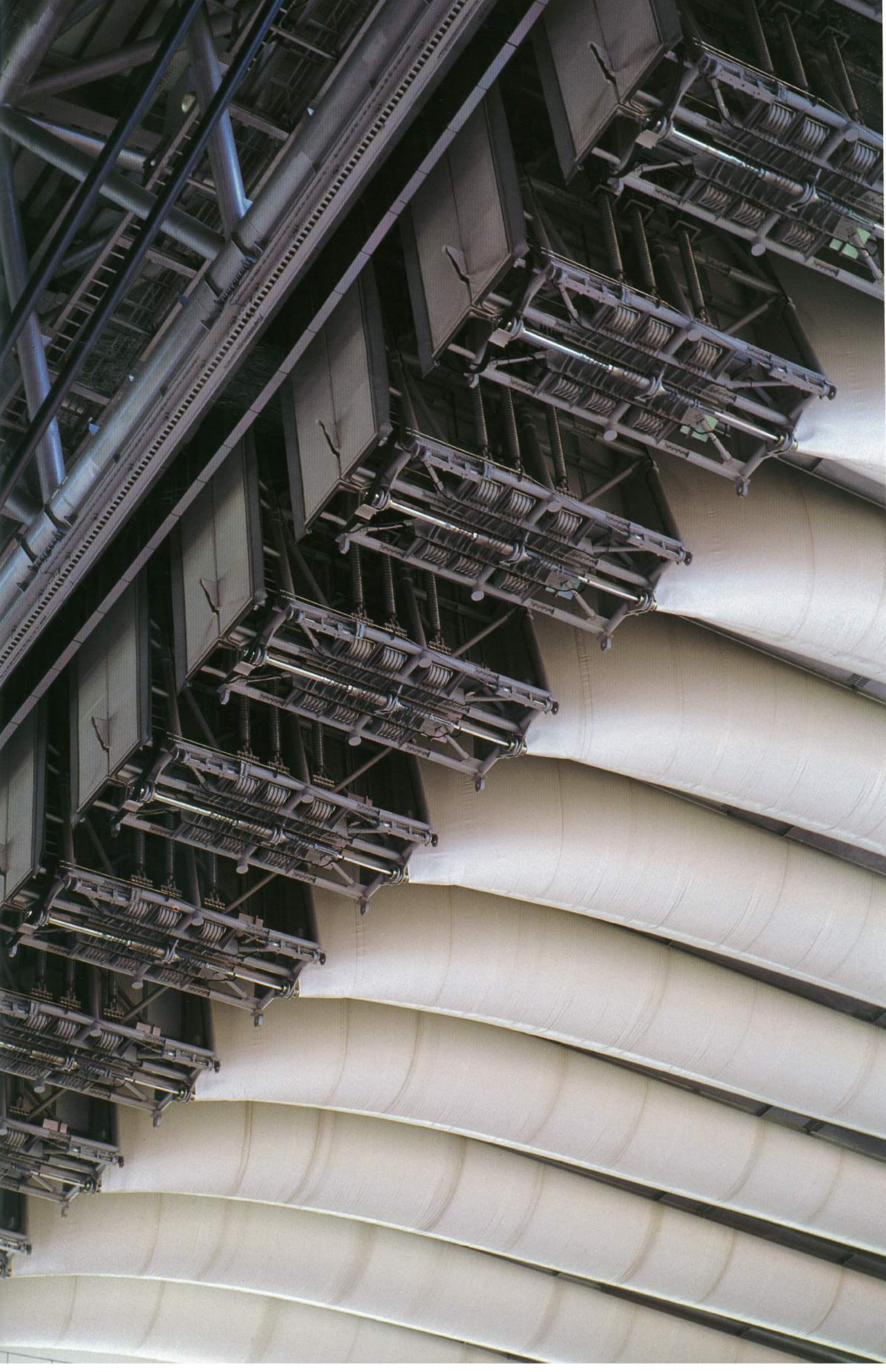
Facing page above: When open, the retractable roof folds into a compact shelter covering the north stand of the stadium. Facing page below: Here the roof is shown in the process of folding. This page: This detail shot shows the moveable trusses in the roof's folded or open position.
