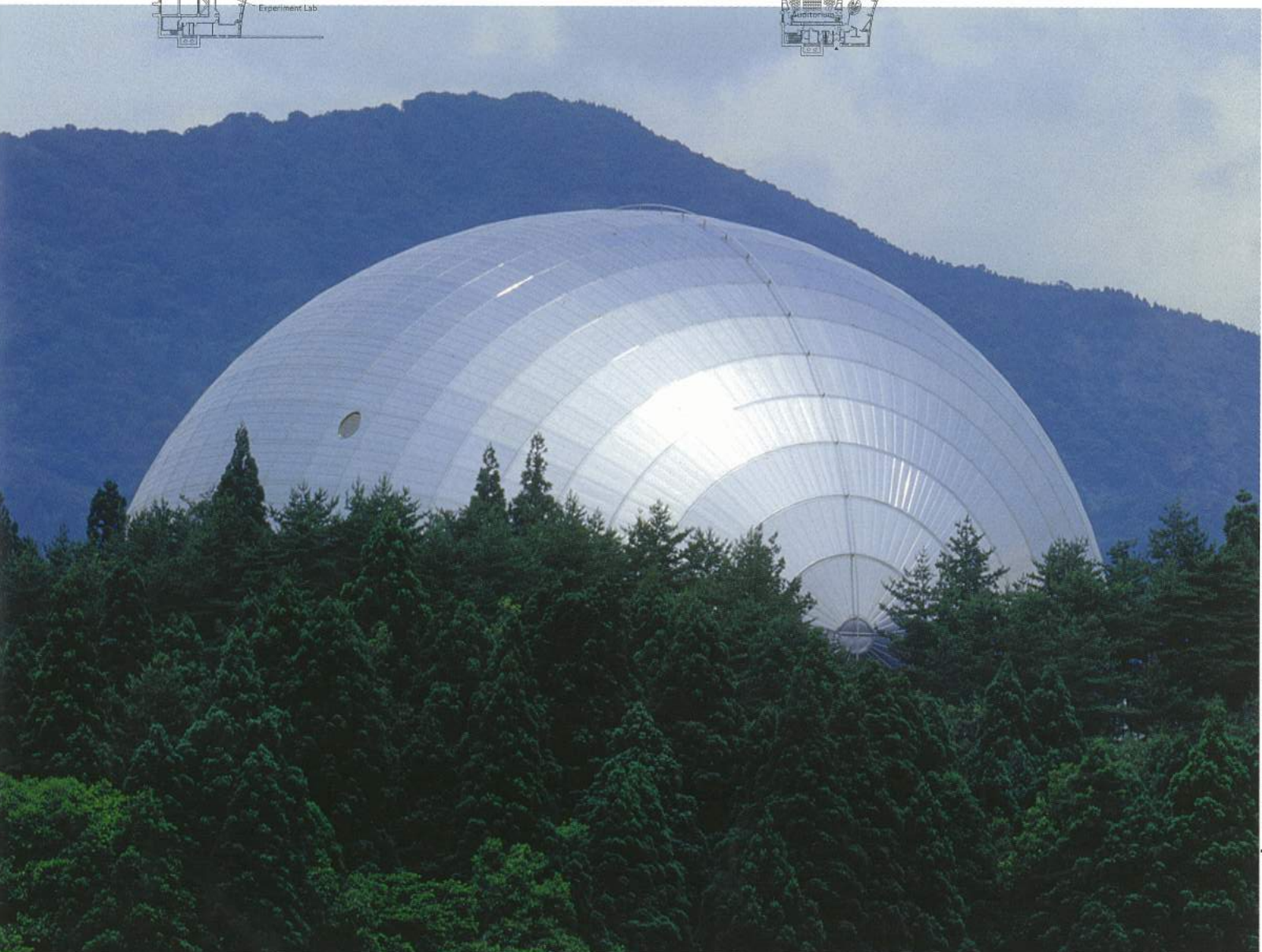
Facing page above: Site plan Facing page below: From the southwest the shining ellipsoid both stands out and blends in with the landscape. This page above: Floor plans This page below: The curve of the exhibition space mirrors the curves of the surrounding mountains.
