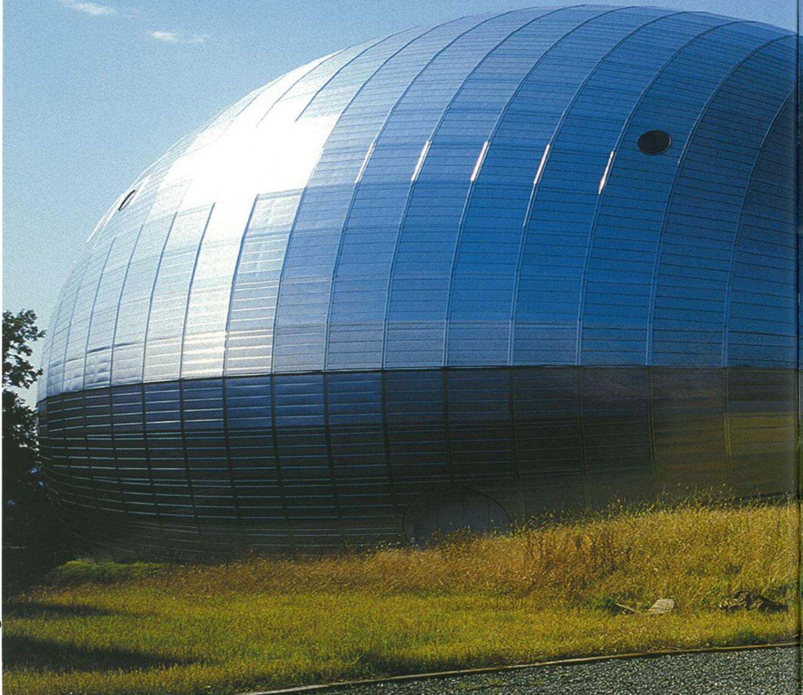
A precast concrete-clad structure adds contrast to the transition between the metallic exhibition hall and the glass curtainwall of the wing building. Inlay: Interior axonometric drawing of the entrance
